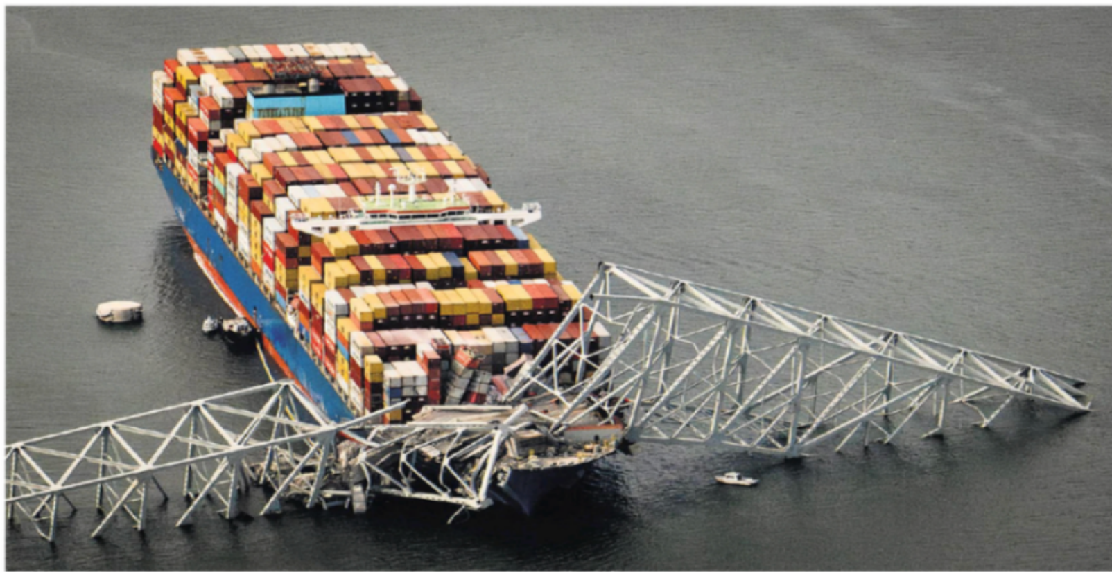
A cargo vessel bound for Sri Lanka caused the Francis Scott Key Bridge in Baltimore to fall on Tuesday, sending construction workers into the water. Two were rescued.
