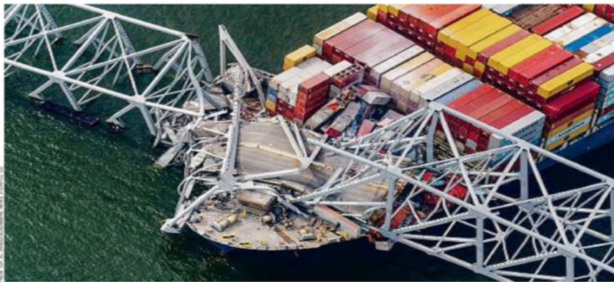
The Francis Scott Key Bridge in Baltimore collapsed (sequence below) after being struck by a ship. Scan a code on A2 for video.
