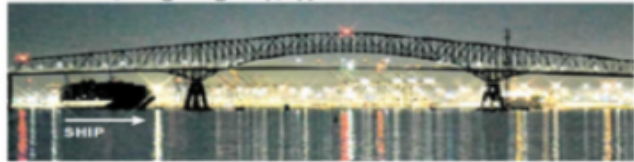
1:27 A.M. The ship changed direction as it neared one of the bridge's piers.
