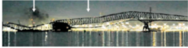
1:28 A.M. The northern span began to collapse seconds later.
