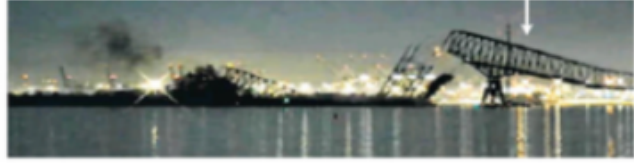
1:29 A.M. Within 30 seconds of impact, the main spans had fully collapsed.
