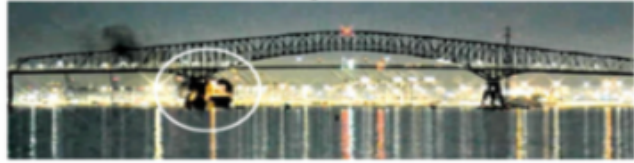
1:28 A.M. Southern and central spans collapsed within seconds of impact.
