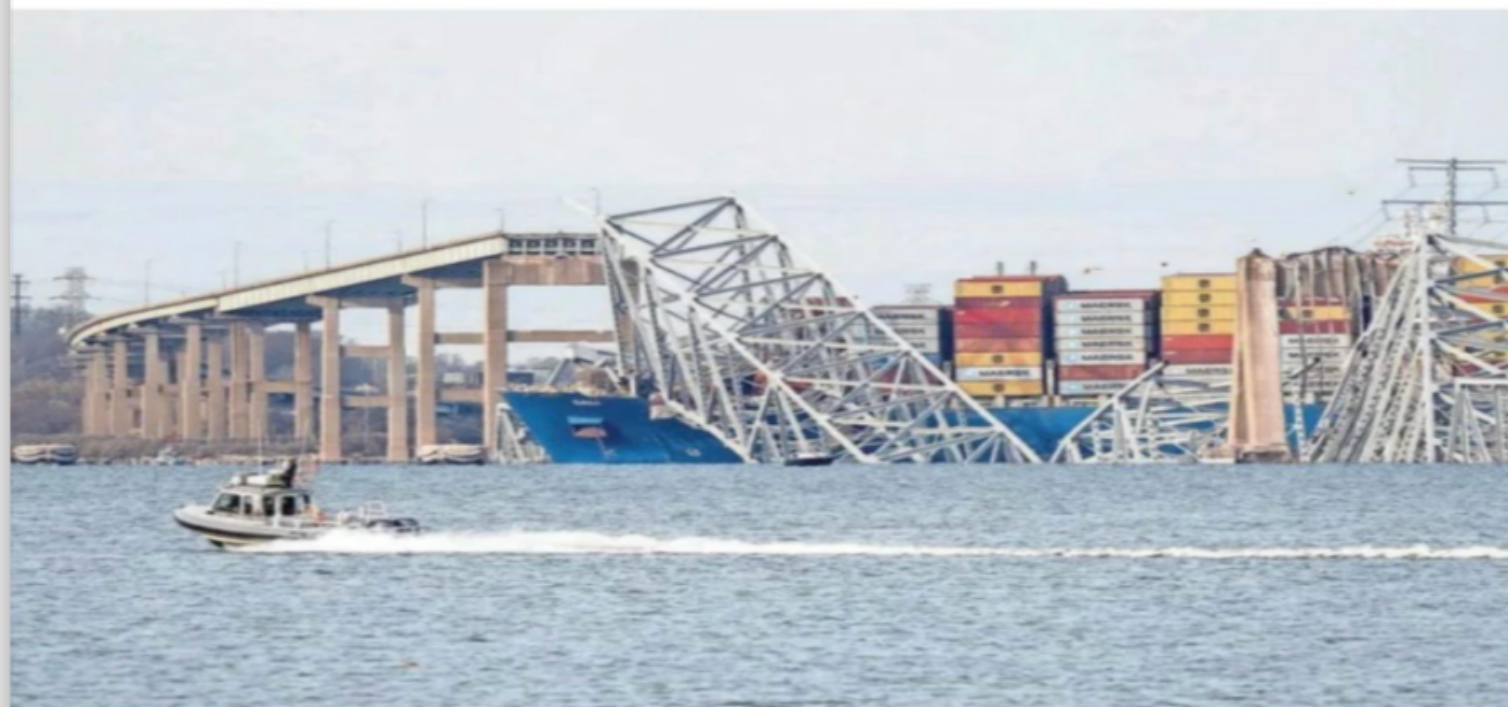
The Francis Scott Key Bridge, a major span over the Patapsco River in Baltimore, collapsed after it was struck by a large cargo ship, prompting a massive emergency response for multiple people in the water. PHOTOS BY JASPER COLT/USA TODAY
